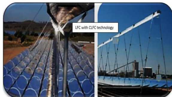
Figure 8. Areva Solar's compact LFC, Kimberlina power station, California [71]
