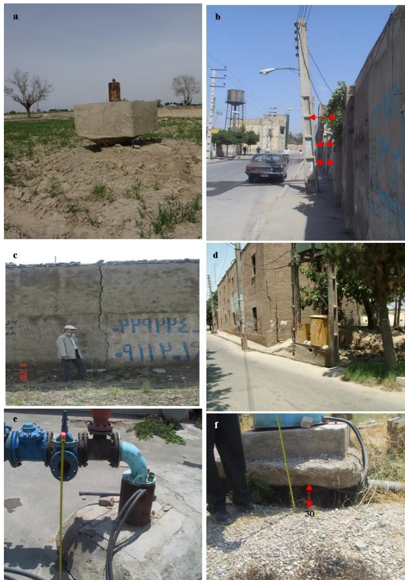
Figure 13: Evidence of progressive land subsidence at southwest of Tehran, a,b) coming up piezometric well and tilting of electrical tower (Sabashahr) ,c,d) cracks in building (Eslamshahr and Ahmadabad) , e,f) coming up well's casing (Shahriyar and Ahmadabad).
