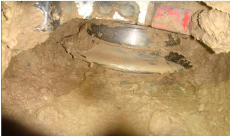
Fig. 10. Clogging of cutting tools due to the presence of ET-5 soil group in the tunnel route of Tehran subway line 7
