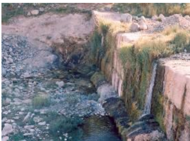
Fig. 5. Rabor Diversion Dam, upstream Diversion Dam was filled with coarse sediments
