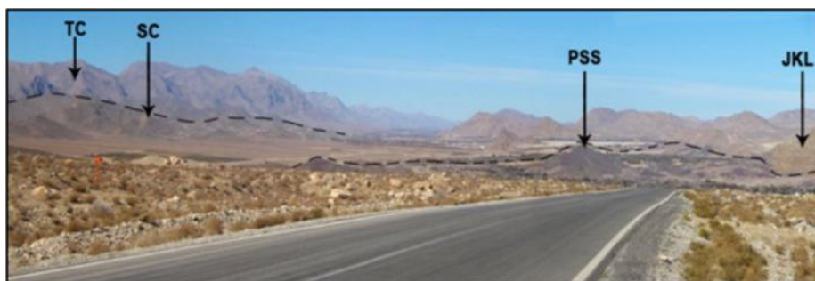
Figure 3. Field relation between Jurassic–Cretaceous limestone (JKL) with purple siltstone (PSS), Surian complex (SC) and Tootak complex (TC) along the Bavanat plains, east village of Monj (view to the west)
