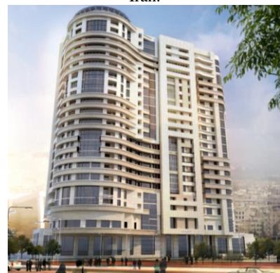
Figure 2. View of Yas residential tower, Mashhad, Iran.
