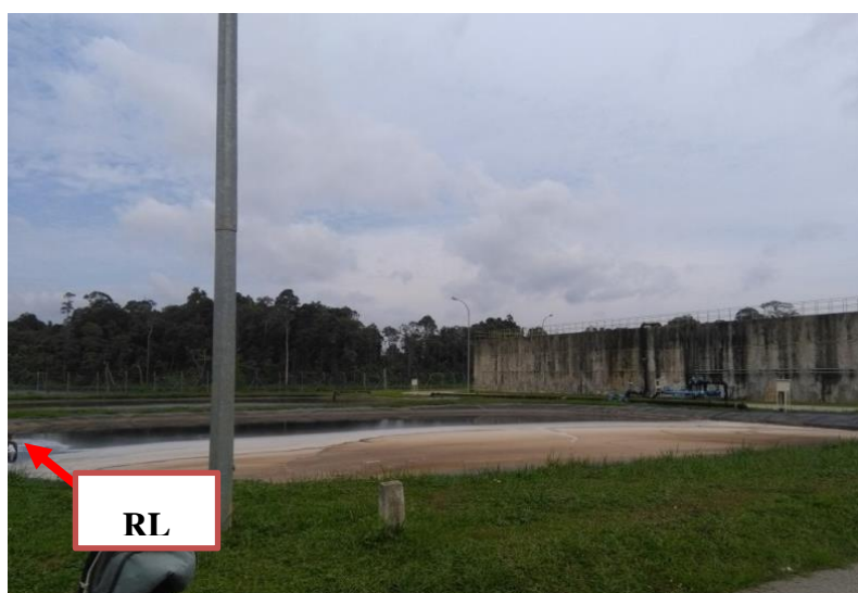
Fig. 2. Raw leachate collected from leachate collection pond
