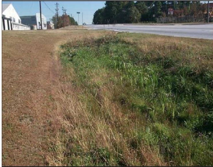
Fig. 9. Implemented vegetative swale (Pennsylvania Department of Environmental Protection Bureau of Watershed Management, 2006)
