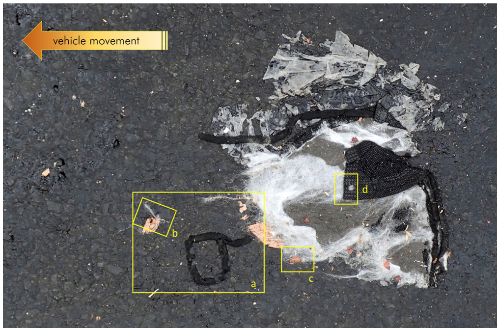
Fig. 4. A single use surgical-type face mask embedded in a bitumen repair patch. The yellow rectangles show the position of the detailed images Figure 5a–d .
