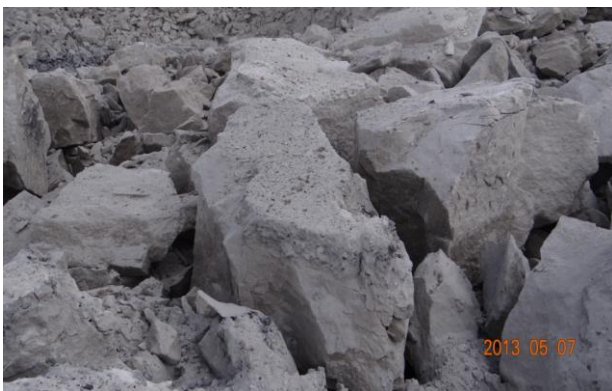
Figure 23. Oversize boulders generated from the top portion of the holes in the trial blast conducted with the decked charge at the 4 th Bench, Quarry No. 2.
