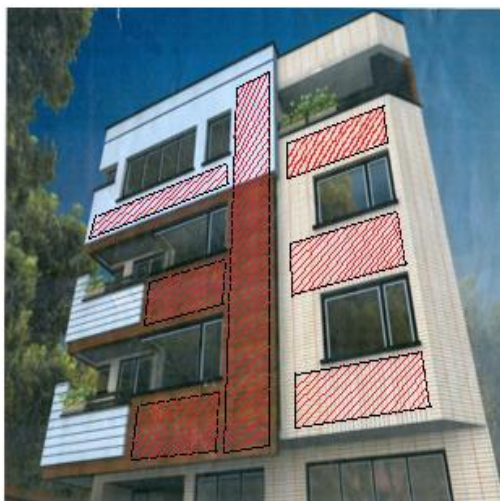
Figure 2. Existing building facades (a: West and b: South), the PV and SWH places of installation are hatched on the Façade
